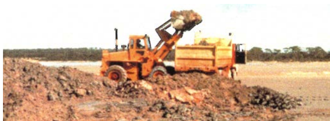
Figure 7: Lake Chandler excavation (Historic photo: Martin Jacobsen, ActivEX Ltd.).
