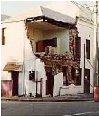
Some of the buildings in Newcastle date back to the 1860s, most of them were either unreinforced masonry (URM) or had URM components such as chimneys, walls, verandahs or access stairs. The proximity of the sea and a large steel works caused widespread corrosion of steel ties between the brick walls or wall and timber frame, and in the suspension ties of awnings and parapets where they existed. As a result all such buildings were highly vulnerable to horizontal shaking.
